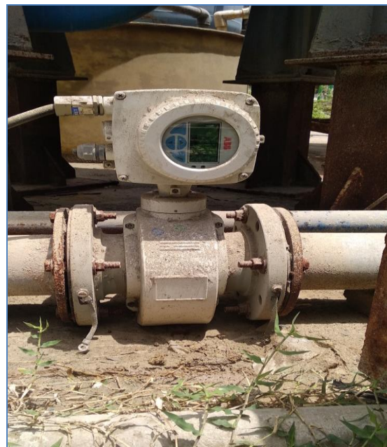
Flow meter for Cement Mill consumption
