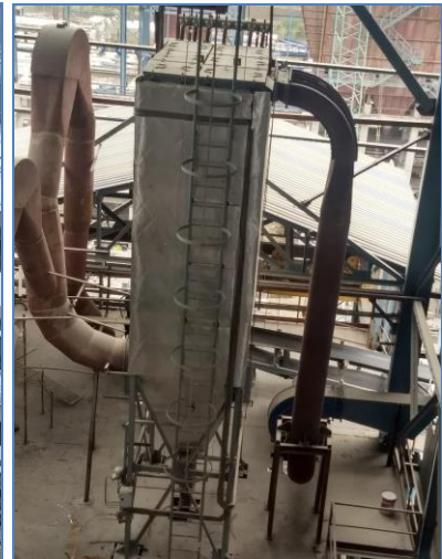
Bag Filters at transfer points
